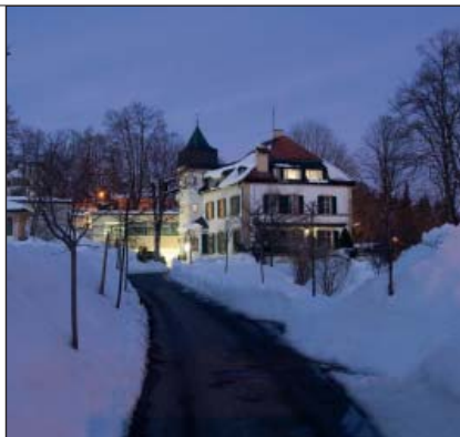
The manufacturing facility in Le Locle.
